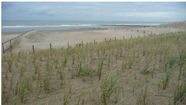
Figure 1 - Marram grass Dune-Dike at Westende, Belgian Coast (photo courtesy: Herman Troch).
