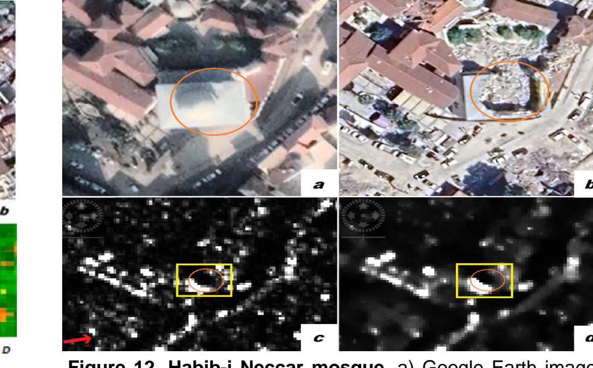
Figure 12: Habib-i Neccar mosque. a) Google Earth image before earthquake, b) Google Earth image after earthquake, c) SAR image, d) Filtered SAR image. Orange circle indicates the area where roof of the mosque is collapsed. (TerraSAR-X Acquisition date : 23 Mar 2023)
