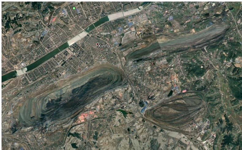
Fushun west open pit mine
